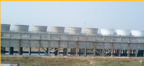
SUPER THERMAL POWER PROJECT AT NAGPUR, MAHARASHTRA
